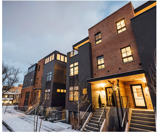
Townhouse | BlockM, Bozeman, MT
